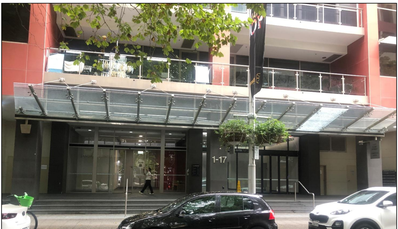
Figure 12 – Ground floor entrance of the subject site. Source (Council Site Inspection)
