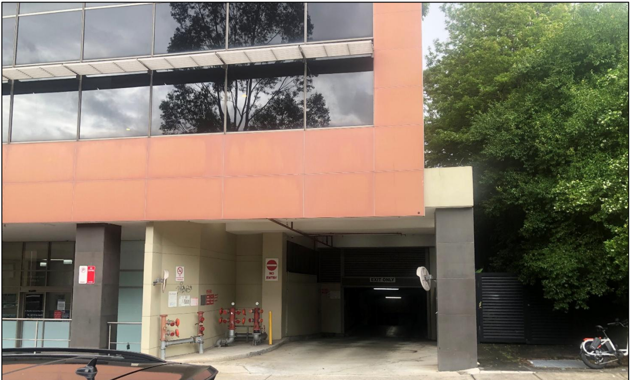
Figure 13 – Basement parking exists on Victoria Street Source (Council Site Inspection)
