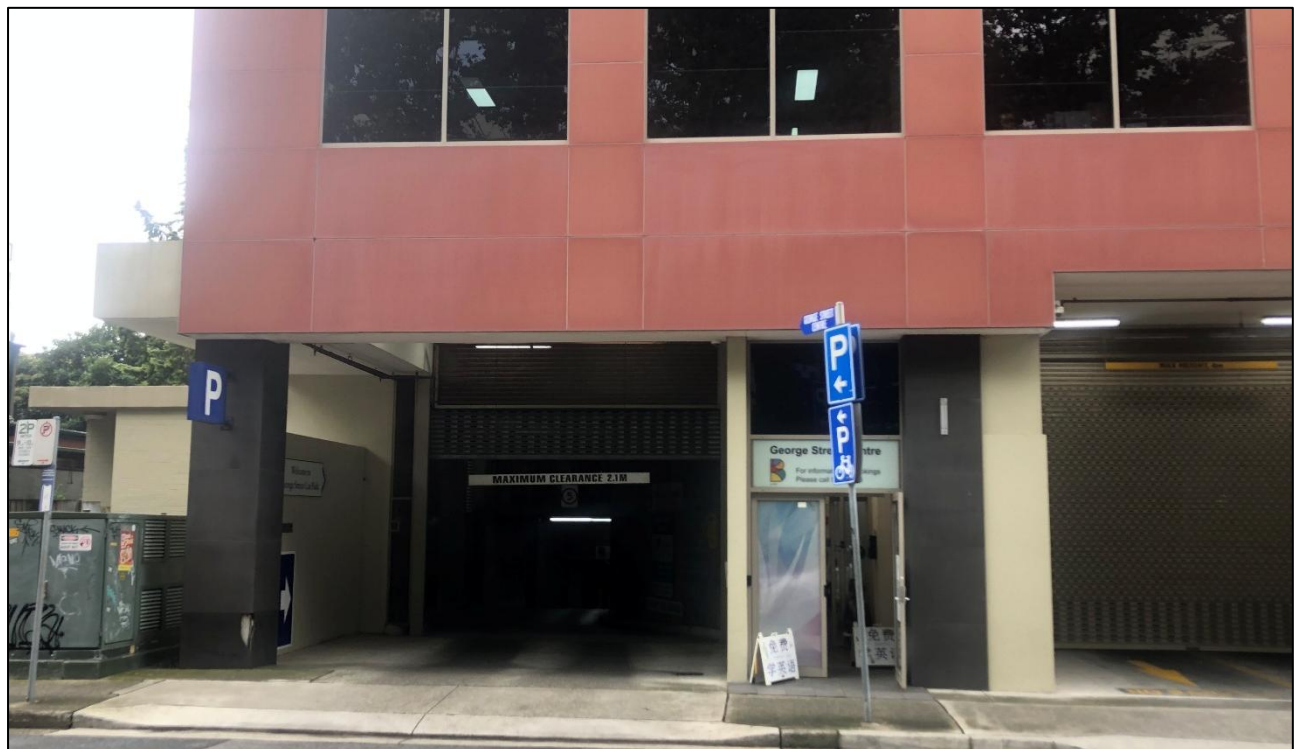
Figure 14 – Basement parking entrance on George Street Source (Council Site Inspection)
