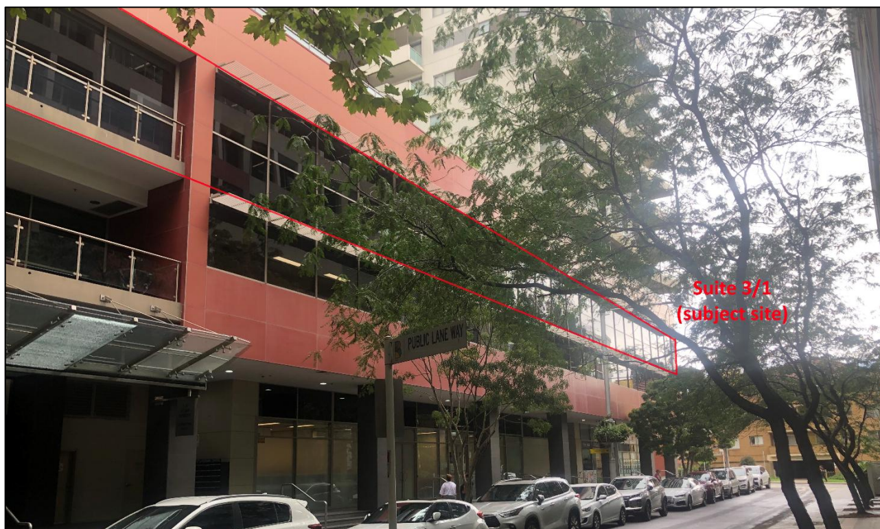
Figure 10 – Elsie Street frontage of the subject site. Source (Council Site Inspection)
