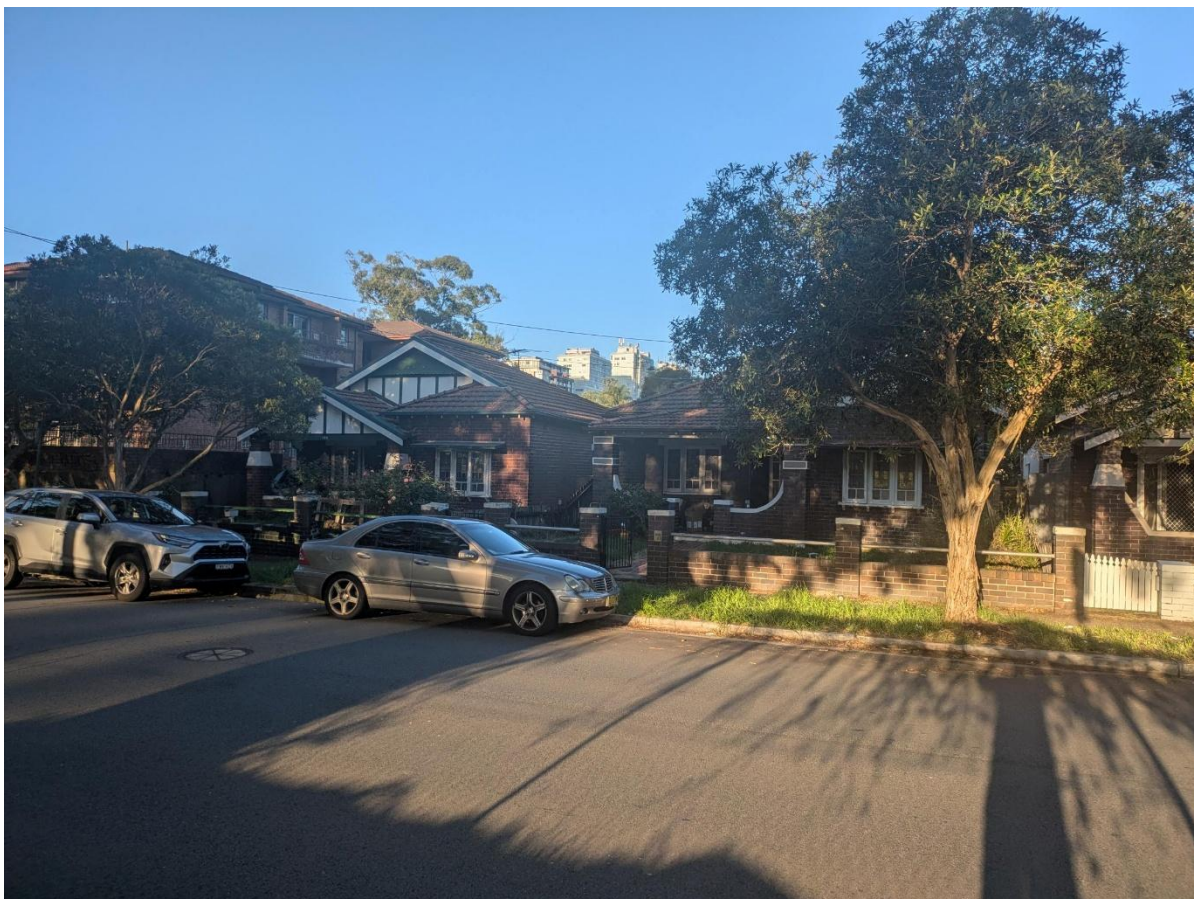
Figure 6: (above) View of the subject site in March 2026 as viewed from Wentworth Road. The two houses in view are proposed to be demolished for the development. Source: Sim (2026).
