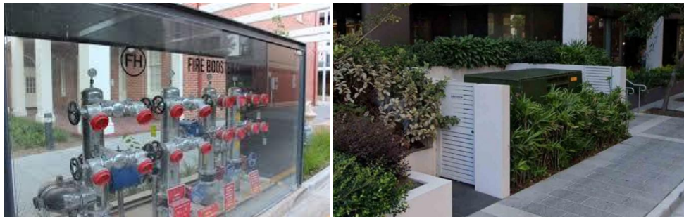
Figure 11: Integration of substation, hydrant & boosters with landscaping and building elements (Source: Google images)
