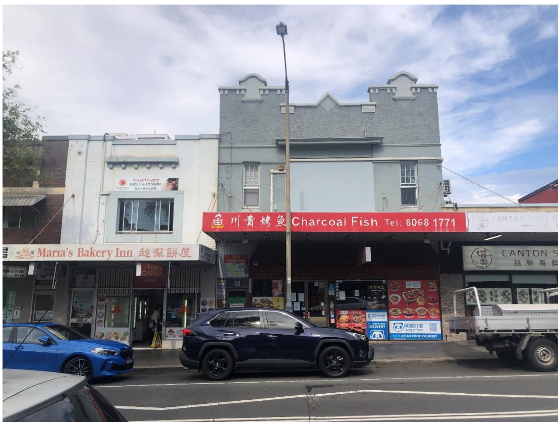
Figure 14: No.242 – 248 Burwood Road, heritage item Federation shops – First Floor Facades located on the east side of the site. Source, site inspection on 18/10/2024
