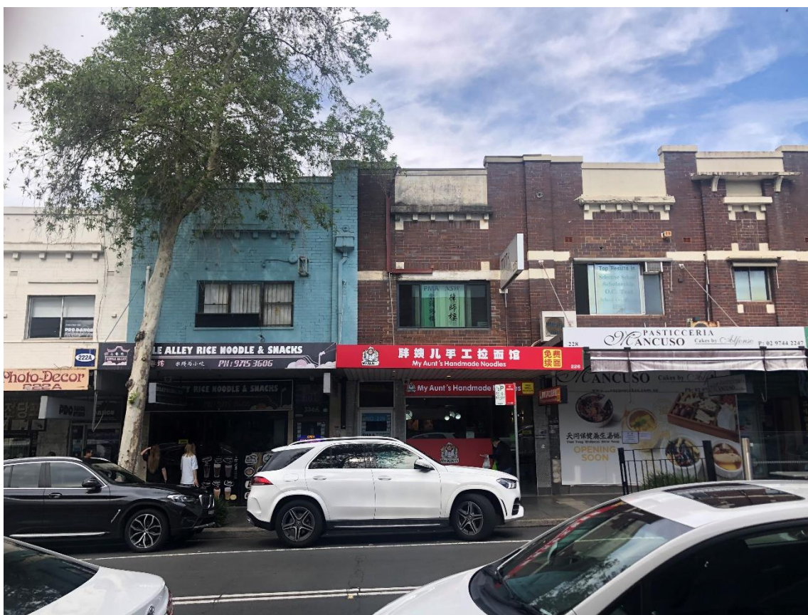
Figure 13: No.224 and 228 – 230A Burwood Road, Burwood, heritage item federation shops – First Floor Facades located on the east side of the site. Source, site inspection on 18/10/2024.
