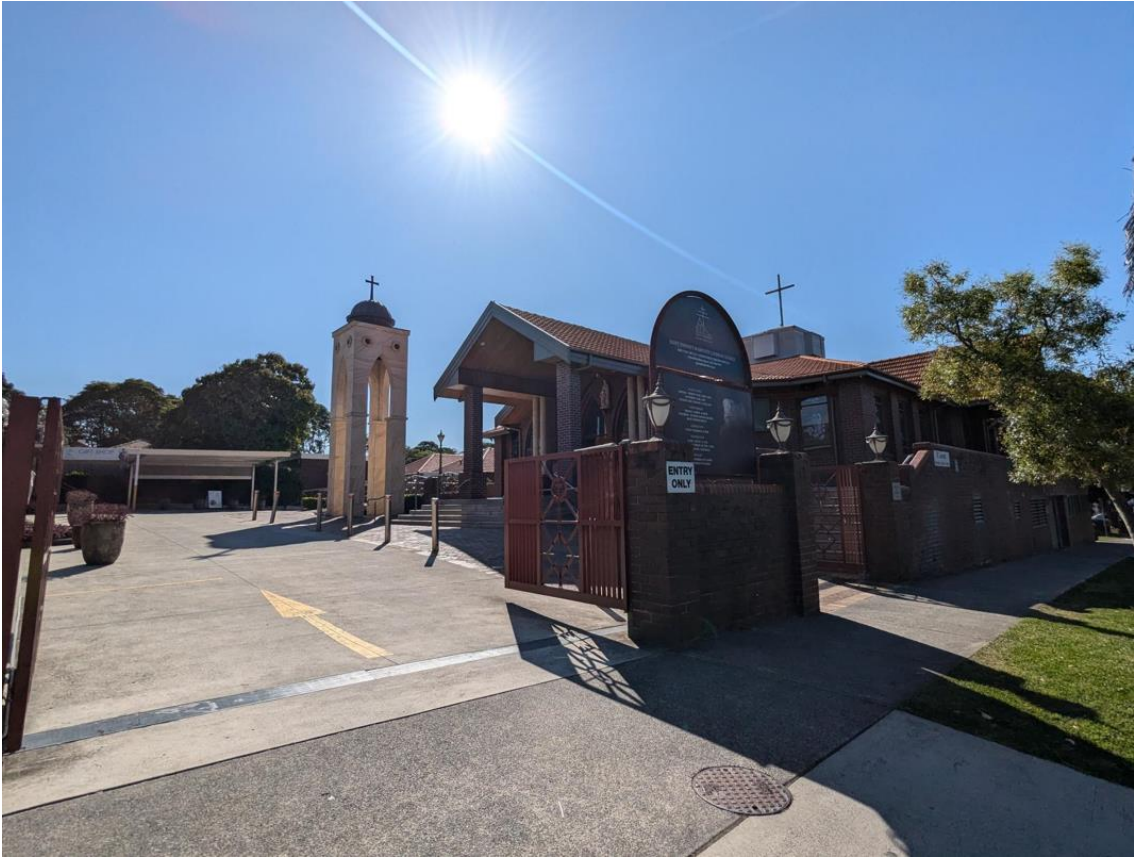
Figure 4 – Church Entrance from Acton Street Source: Council Site Inspection
