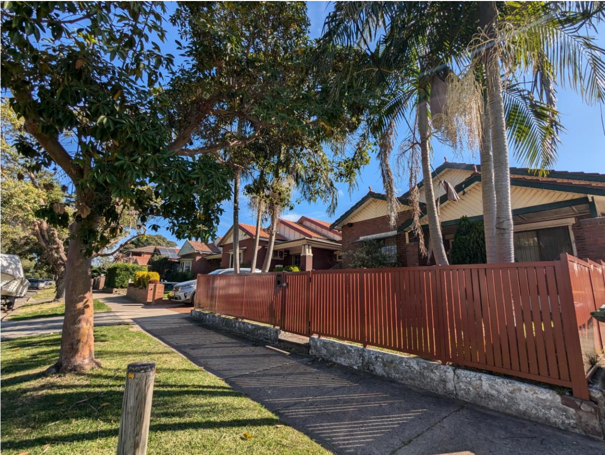
Figure 5 – No. 11 Acton Street (right) to be demolished as part of the development to provide the new youth kitchen, library and associated landscaping. Source: Council Site Inspection
