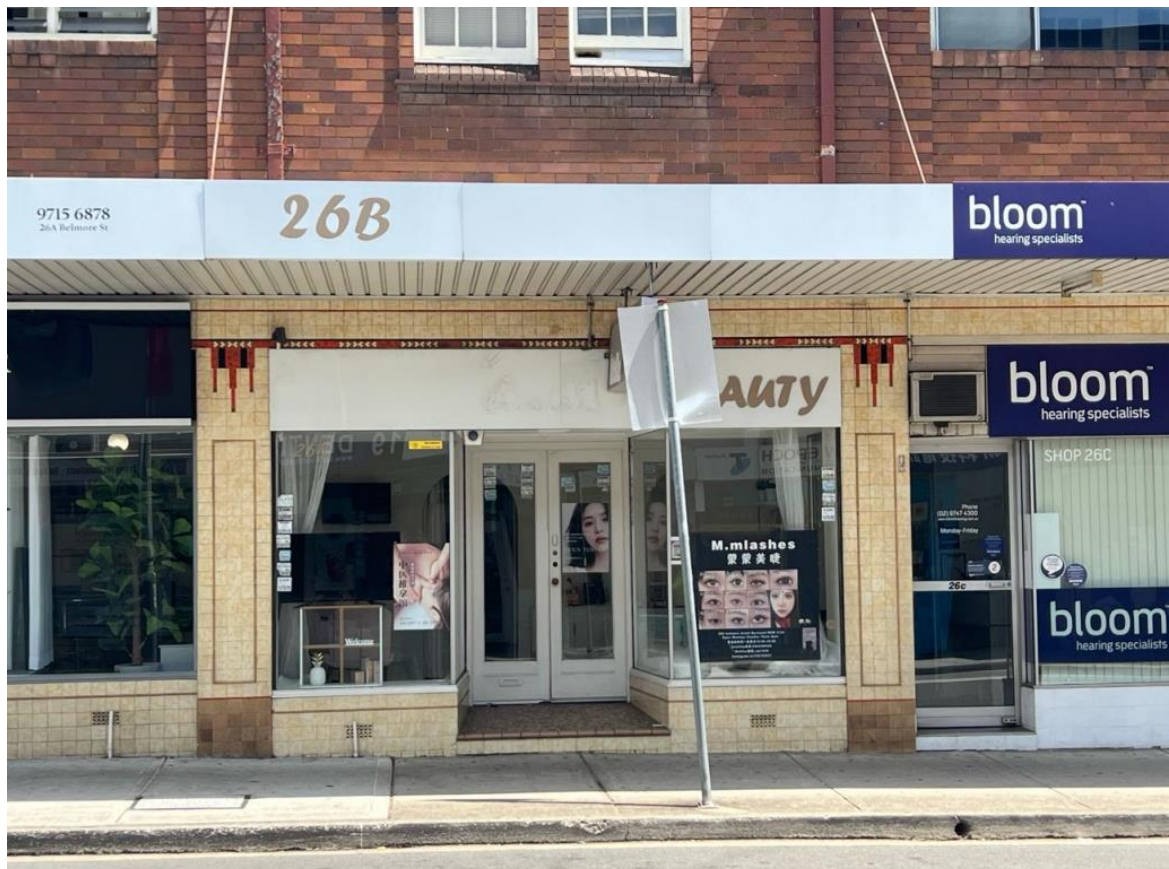
Figure 8: The subject shop frontage of the Development Application, viewed from Belmore Street. Extracted from the Heritage Impact Statement prepared by Touring the past, dated 06/08/2024.
