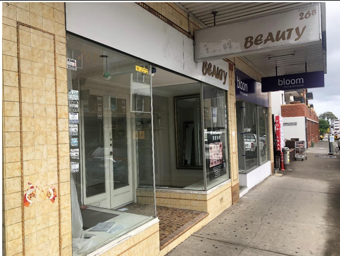
Figure 9: The subject shop frontage and existing under awning sign. Source, site inspection on 14/10/2024
