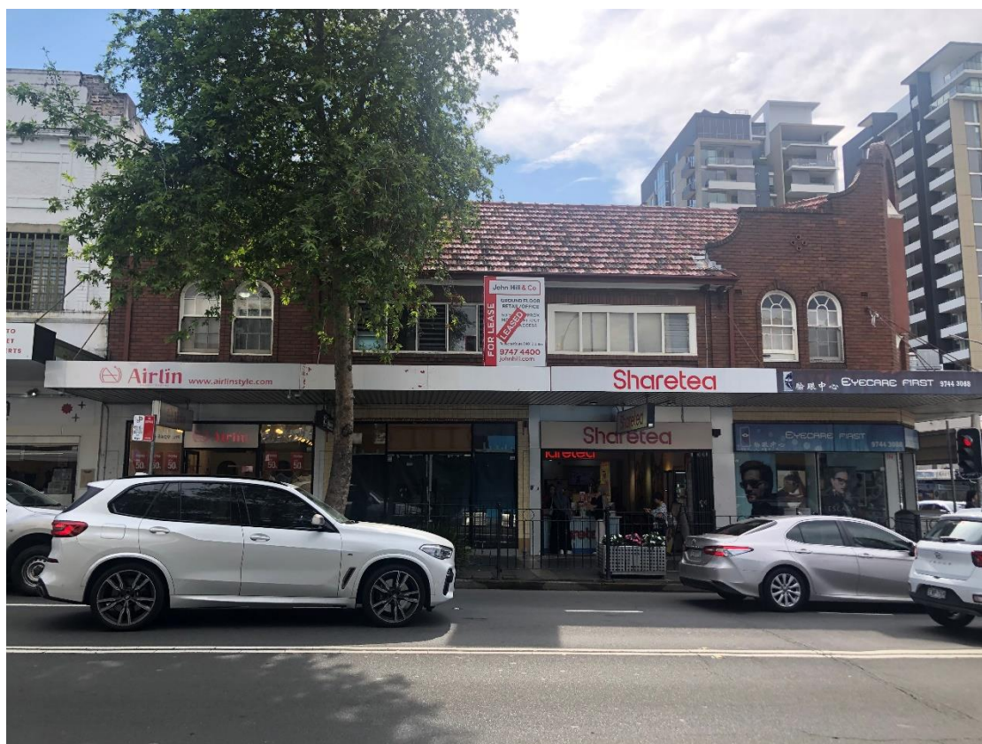
Figure 12: Burwood Road frontage. Source, site inspection on 18/10/2024.
