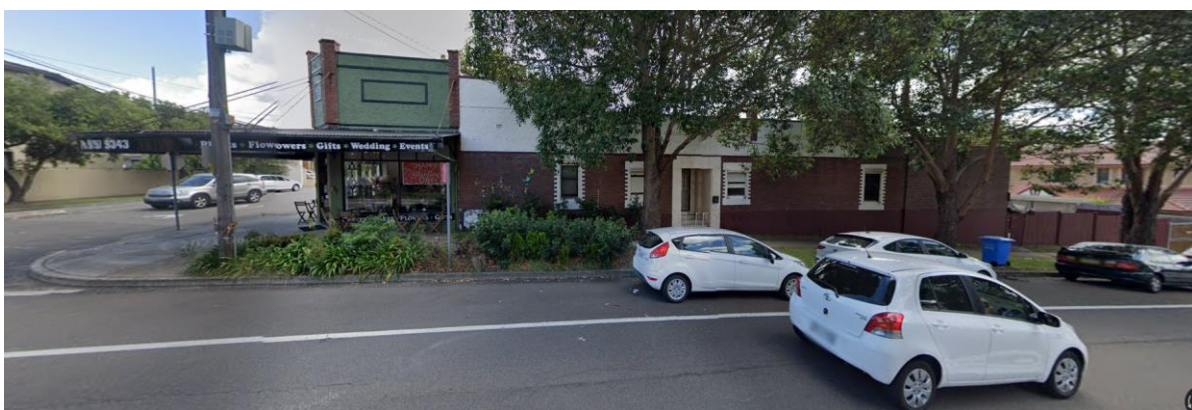
Figure 3: Existing southern façade facing Arthur Street (Source: Google Maps).
