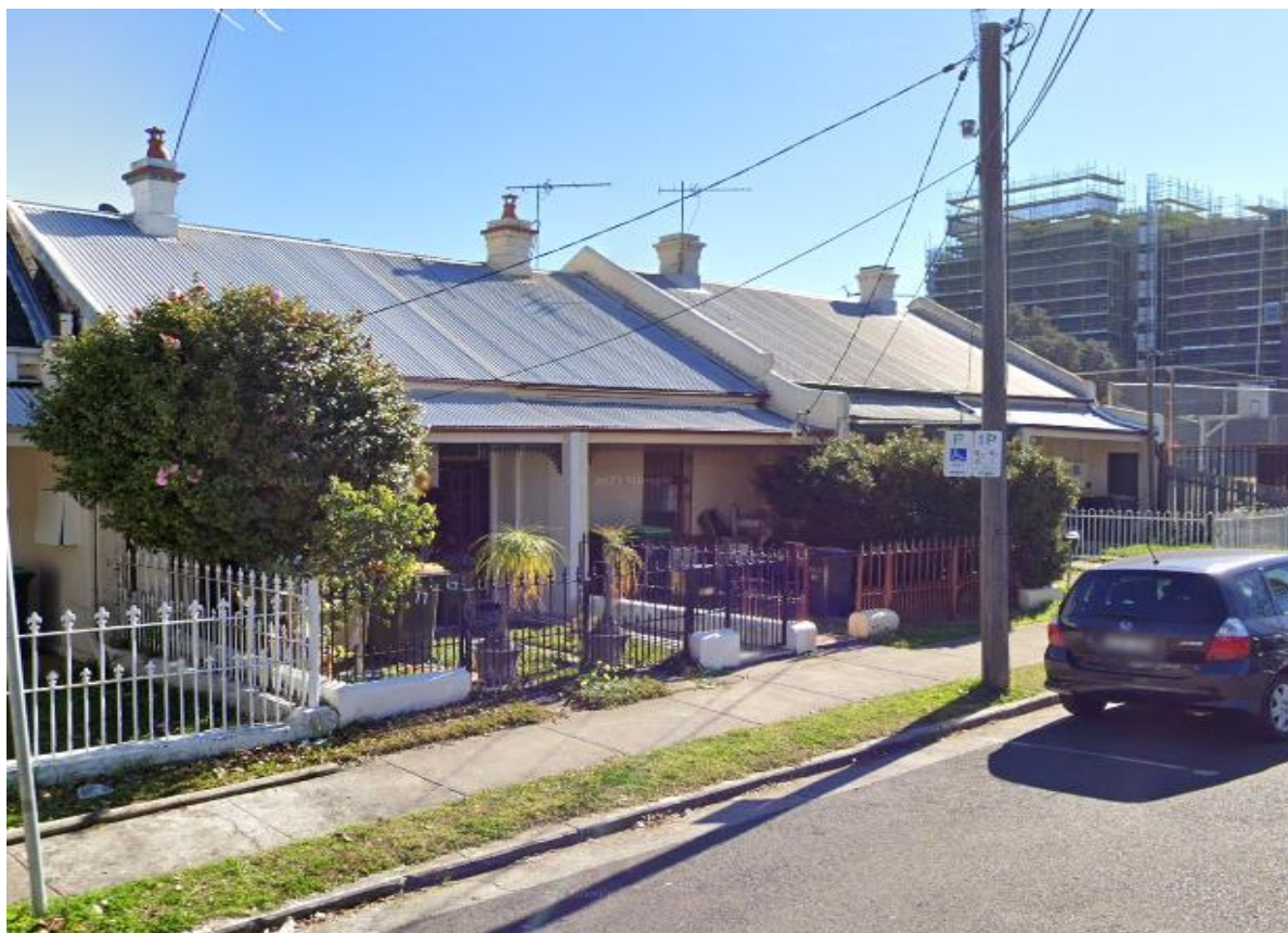
Figure 25 – No. 11,13-15 and 17 Stanley Street, located to the north of the subject site. (Source: Google Maps)
