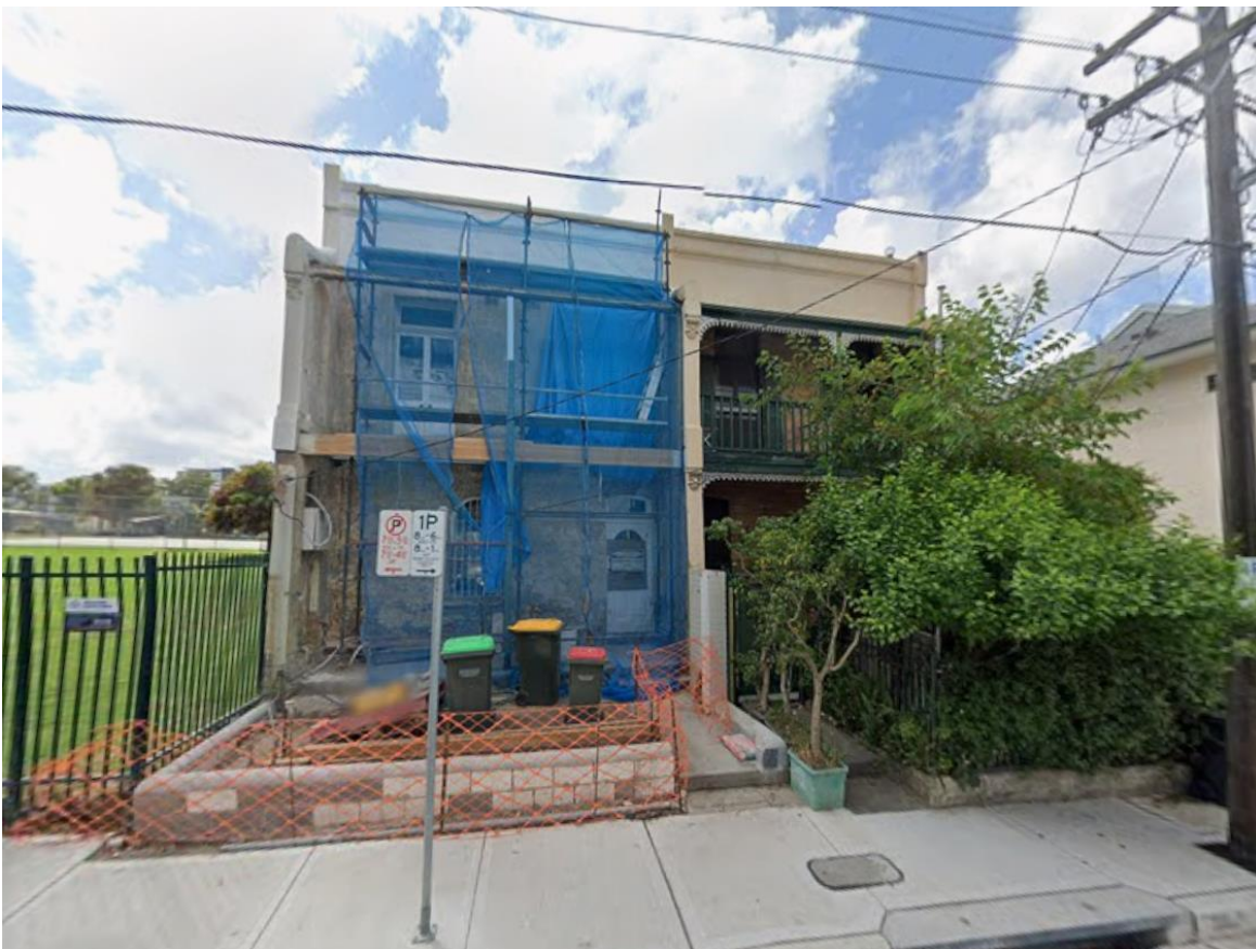
Figure 24 – No.34-36 Oxford Street, located to the west of the subject site. (Source: Google Maps)
