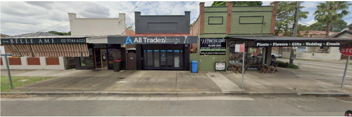
Figure 4: Existing western façade facing Claremont Road (Source: Google Maps).
