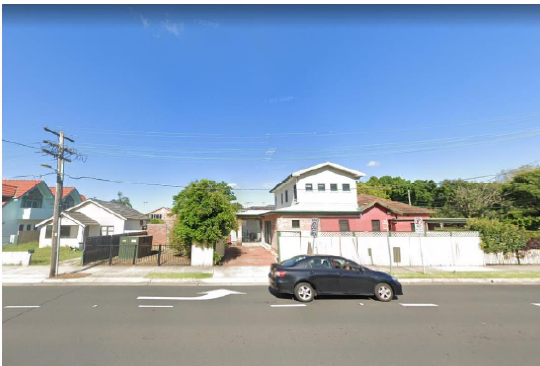
Figure 5 – Streetscape to the north of the site
