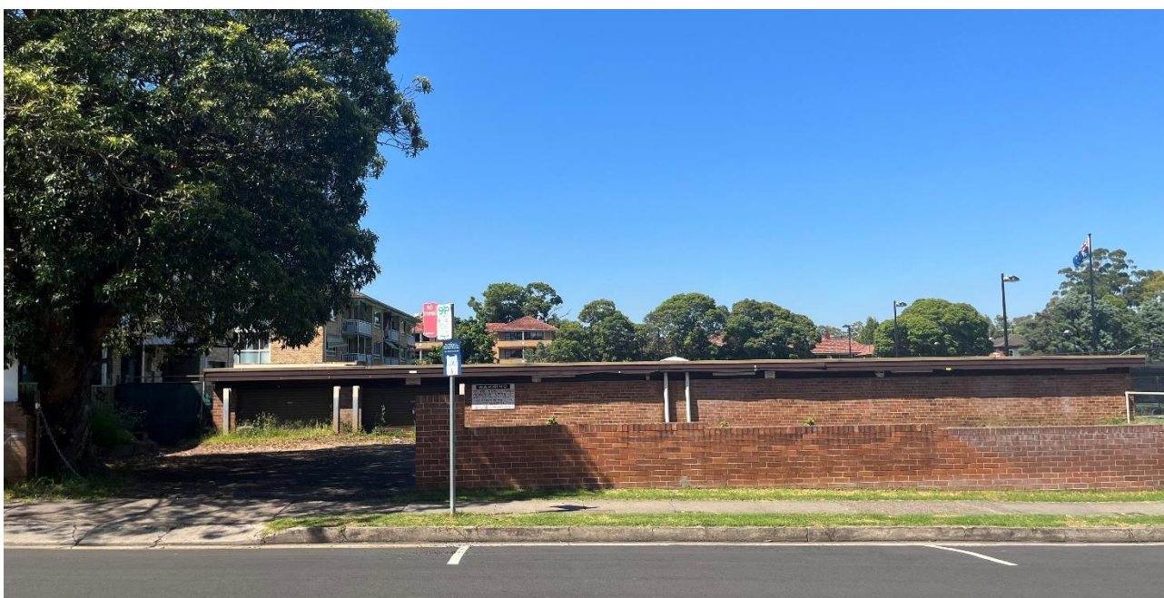
Figure 7: Tennis court car park, viewed to south from Lyons St
