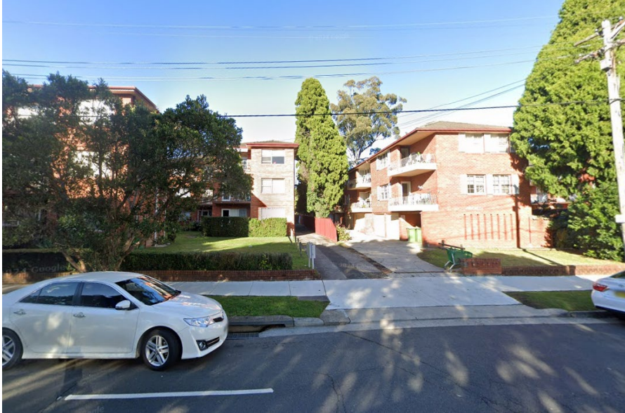
Figure 4: Site view looking South
