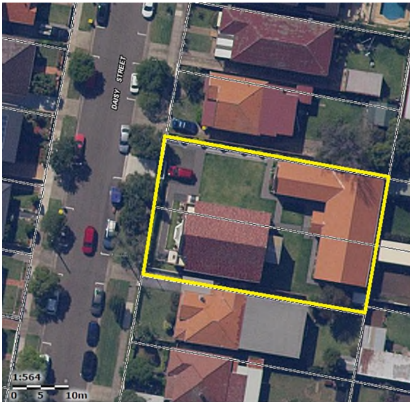
Figure 1: Aerial view of the site at 10 Daisy Street (Source: https://maps.six.nsw.gov.au/ )
