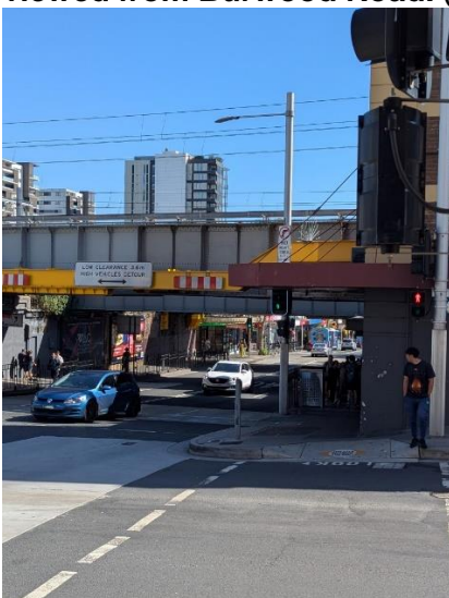
Figure 4: North of the Westpac Building, viewed from Railway Parade. (24/02/2025)
