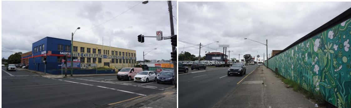
Figure 5 Site Photos – Salvos Site (left), Hoarding to Paramatta Road (right)
