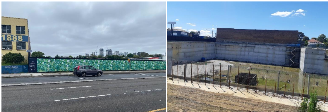
Figure 7 Parramatta Road Frontage (left), existing site excavation (right)
