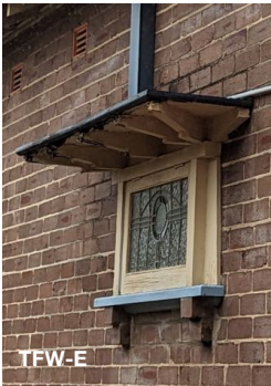
Existing Windows Repair timber framed windows, provide new external hood where required
