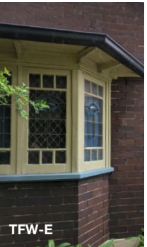
Existing Windows Repair timber framed windows, provide new external hood where required
