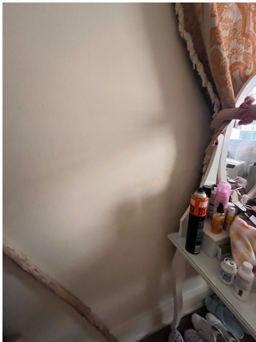
Figure 36 - Unit 6 internal bedroom wall with moisture ingress visible (Source: Three + One Heritage, 2024)
