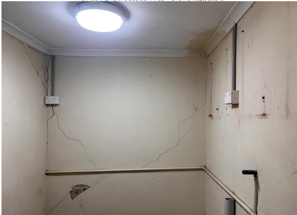
Figure 34 – Interior of rear detached garage, large cracks visible( Source: Three + One Heritage, 2024)
