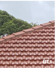
Existing Roof, replace terracotta where required
