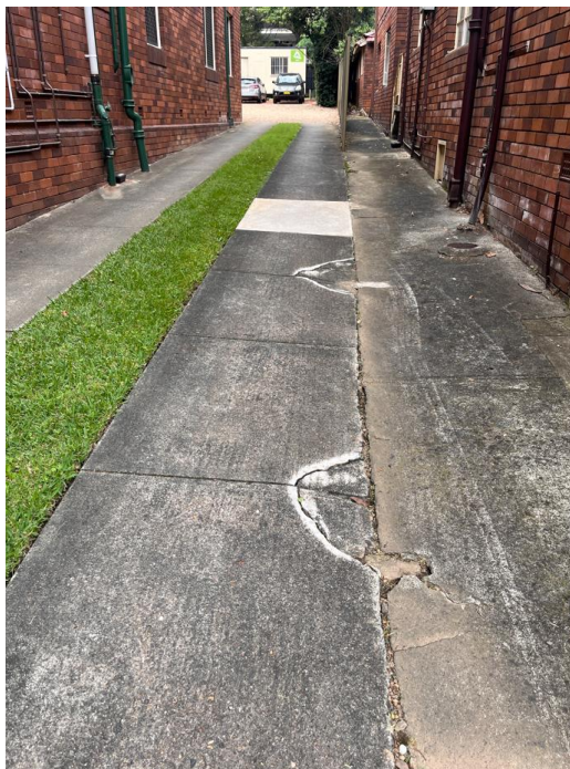
Figure 22 – Side driveway looking south, damage to concrete visible (Source: Three + One Heritage, 2024)
