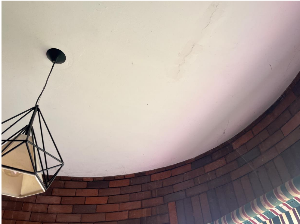
Figure 35 – Soffit of balcony above Unit 2 with cracking visible (Source: Three + One Heritage, 2024)
