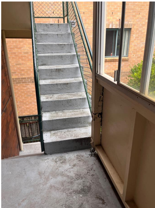
Figure 28 – Rear semi-enclosed balcony, rotted timber visible (Source: Three + One Heritage, 2024)
